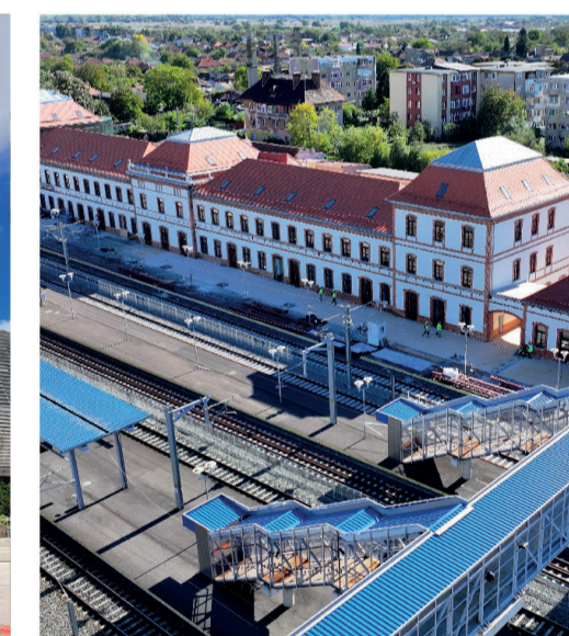
Andreea Tecşa Modernization of railway sections. Pan-European Corridor. Simeria Station. Romania.
