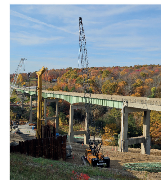
Máximo Serrano Major bridge P3 project. Pennsylvania.
