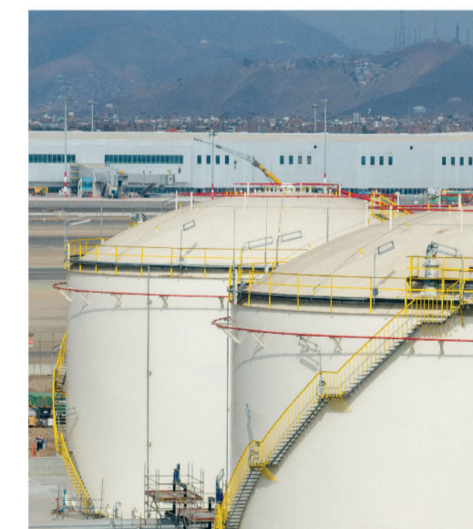
Wilfredo Guerra Expansion of industrial facilities, Lima Airport. Peru.
