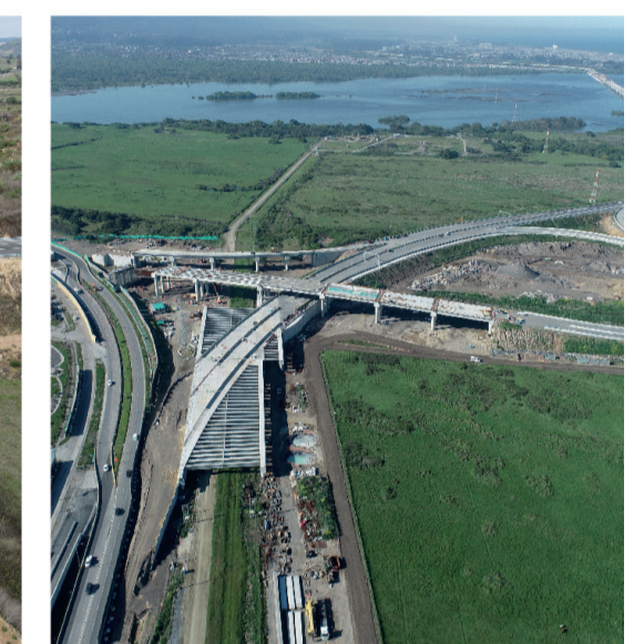
Rodrigo Guerrero Industrial Bridge. Chile.
