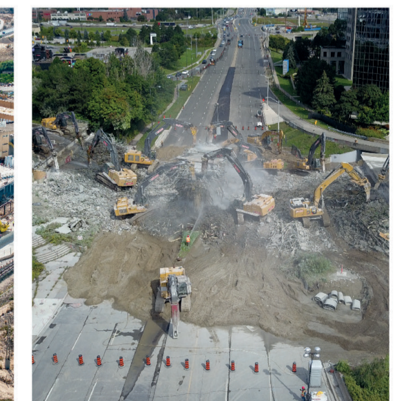
FCC/STC Team Scarborough Subway Extension. Canada.
